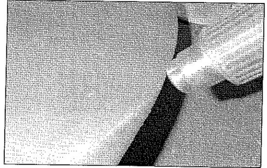
2) Heat with a paint burner the edges of the damaged part till PE softening
