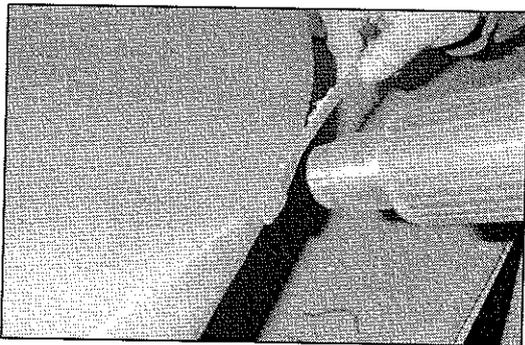
3).Position a tip of a PE strip on the crack then heat it till softening.
