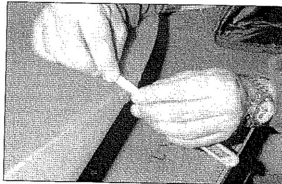
5) Finish spreading with a cutter and scraping off the excess of PE.
