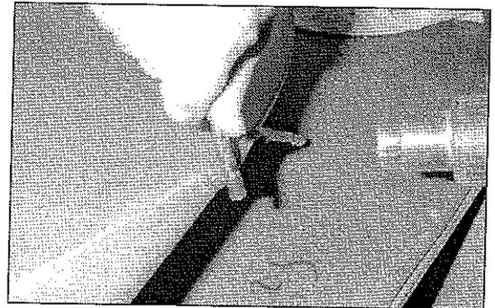
4) Spread progressively the strip on the crack length.
